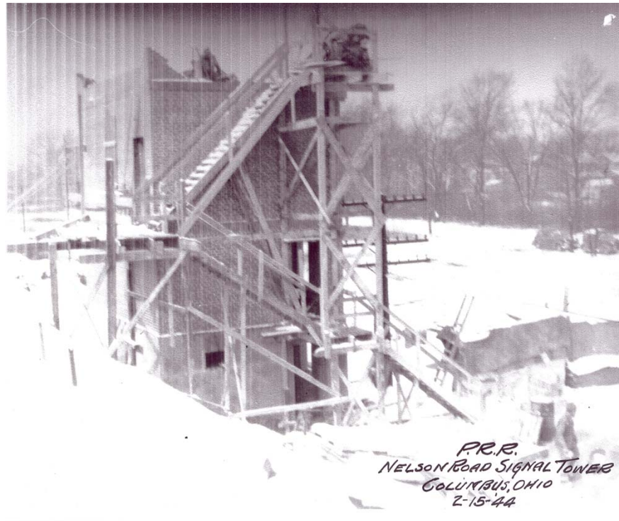
Figure 4 – February 15 and the second floor is bricked up. Cold and snow are not stopping the work.
