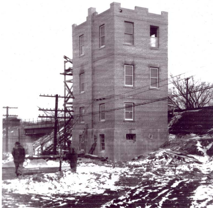
Figure 6 – March 1, the view from the other side looking southeast. The Nelson Road underpass is in the background. Alum Creek is about 1000' to the east.
